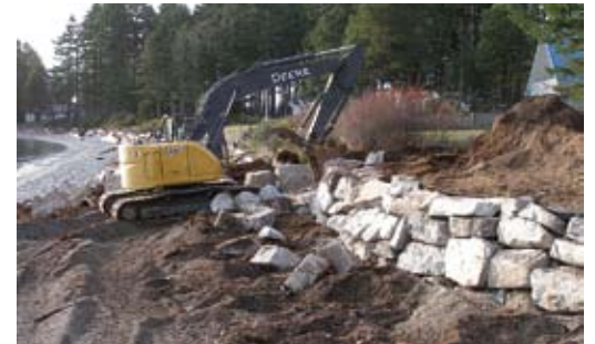
Retaining wall at Palm Beach Regional Park
