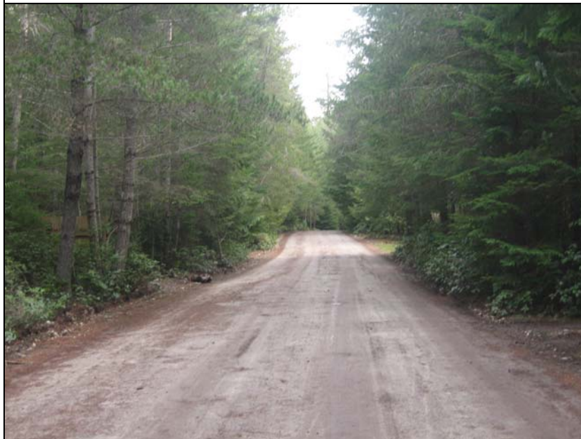
Looking westbound, between Patricia Crescent and S Curve
